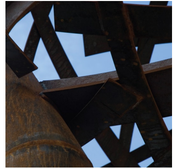
Detail view of the complex welded angles
