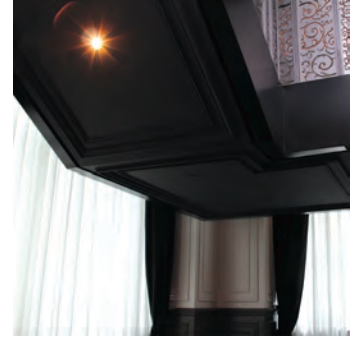
Stringer close out panels with built in lights
