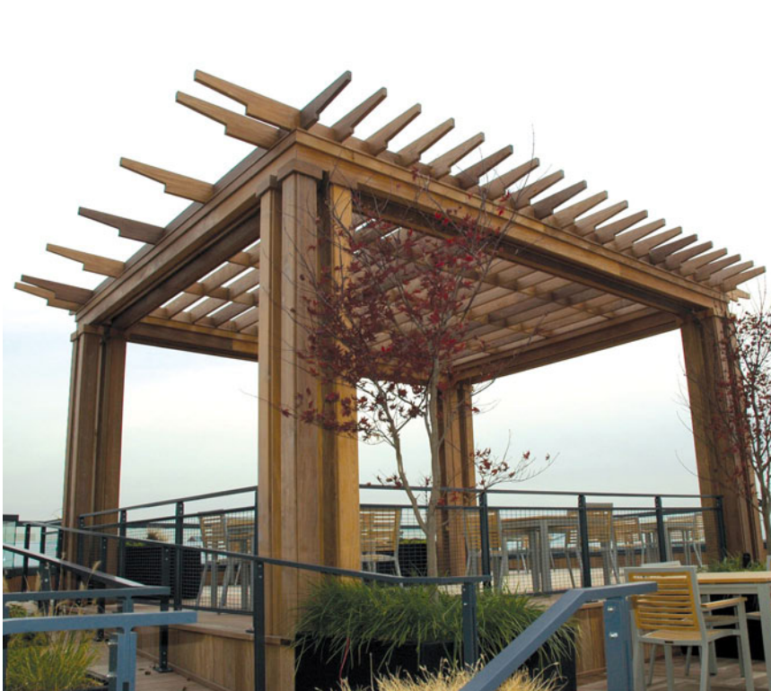
Rooftop railings surround the entire space
