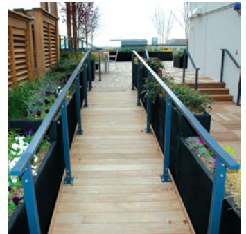
Ramp and stair handrails
