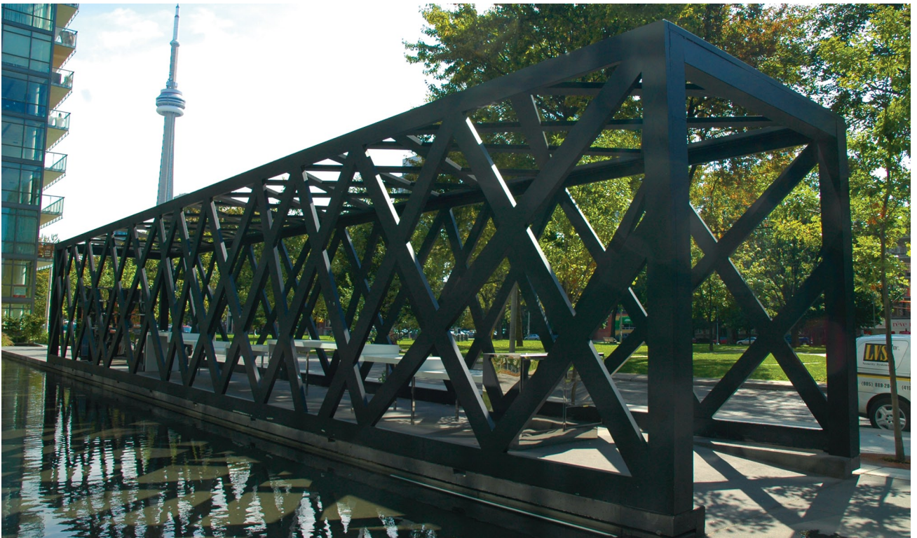
The trellis pavilion at 550 Wellington Ave
