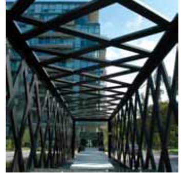
Looking into the trellis pavilion
