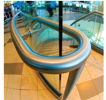
Stainless steel rolled and formed railing detail
