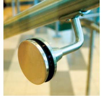
Railing support detail
