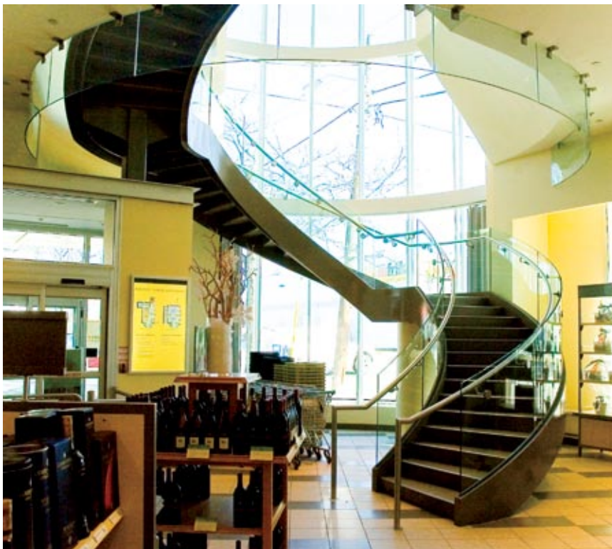
Two story steel and glass spiral staircase with intermittent landings
