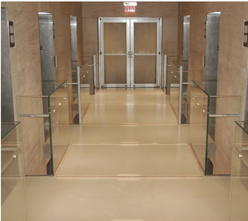
Glass bridge services elevator entrances
