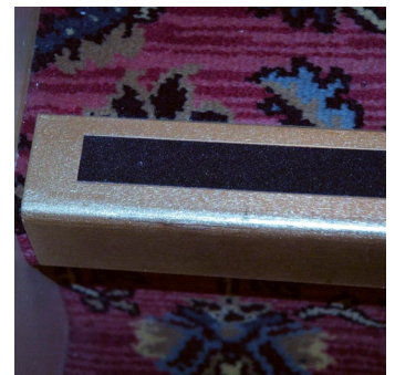
Detail of abrasive non-slip tape
