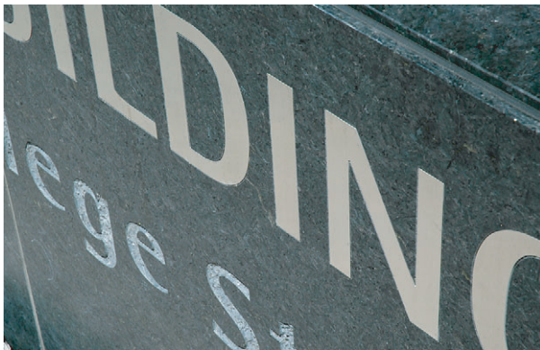
Waterjet cut, brushed stainless steel graphics incised into 1-1/4" thick granite
