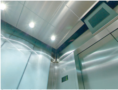
Brushed st. stl. ceiling with recessed pot lights and 'Captive Network' ready monitor
