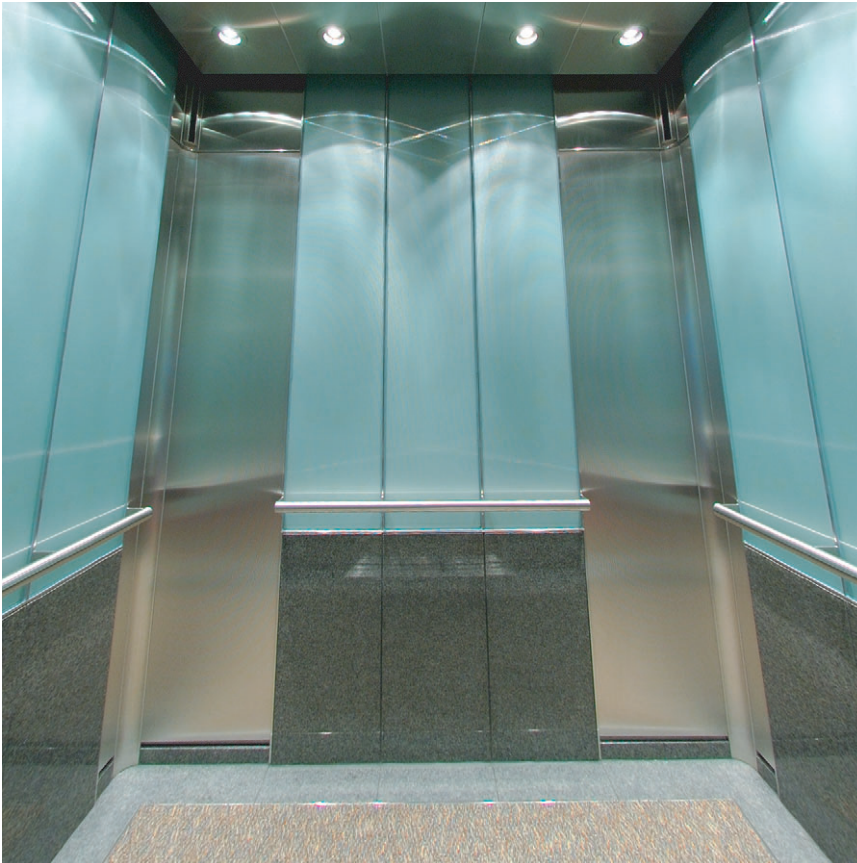
Elevator cab with back-painted reeded tempered glass, granite walls and floor panels and st. stl. handrails with no visible fasteners
