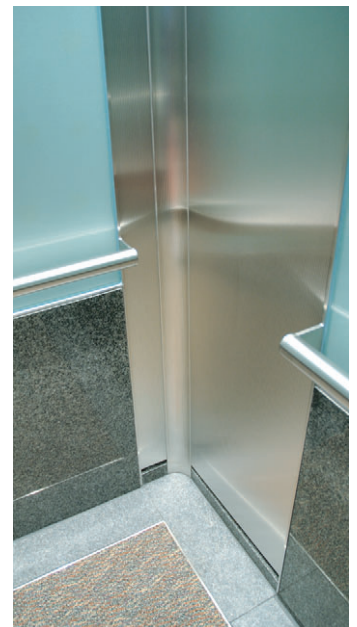
Rigidized st. stl. COP panels and st. stl. handrails with no visible fasteners
