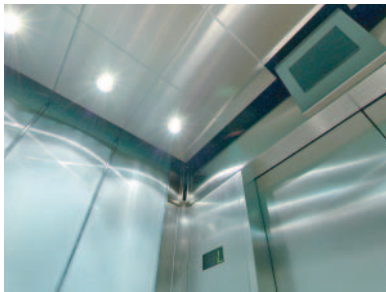
Brushed st. stl. ceiling with recessed pot lights and 'Captive Network' ready monitor
