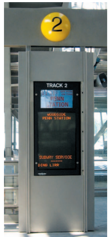
Stainless steel cladding and LED signboard
