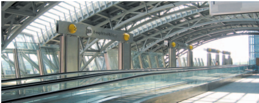
Array of girders spanning approximately 150 feet
