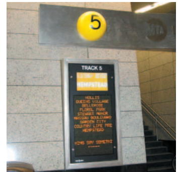
Spun and painted metal globe atop LED signboard
