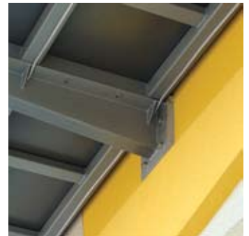
(31) outriggers connected to building column
