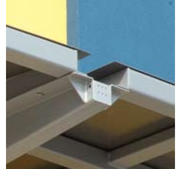
Eavestrough detail, prior to final cladding
