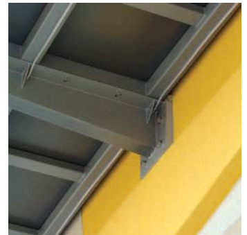
(31) outriggers connected to building column
