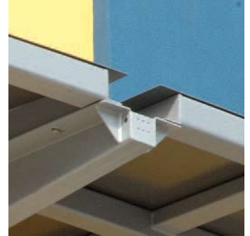
Eavestrough detail, prior to final cladding
