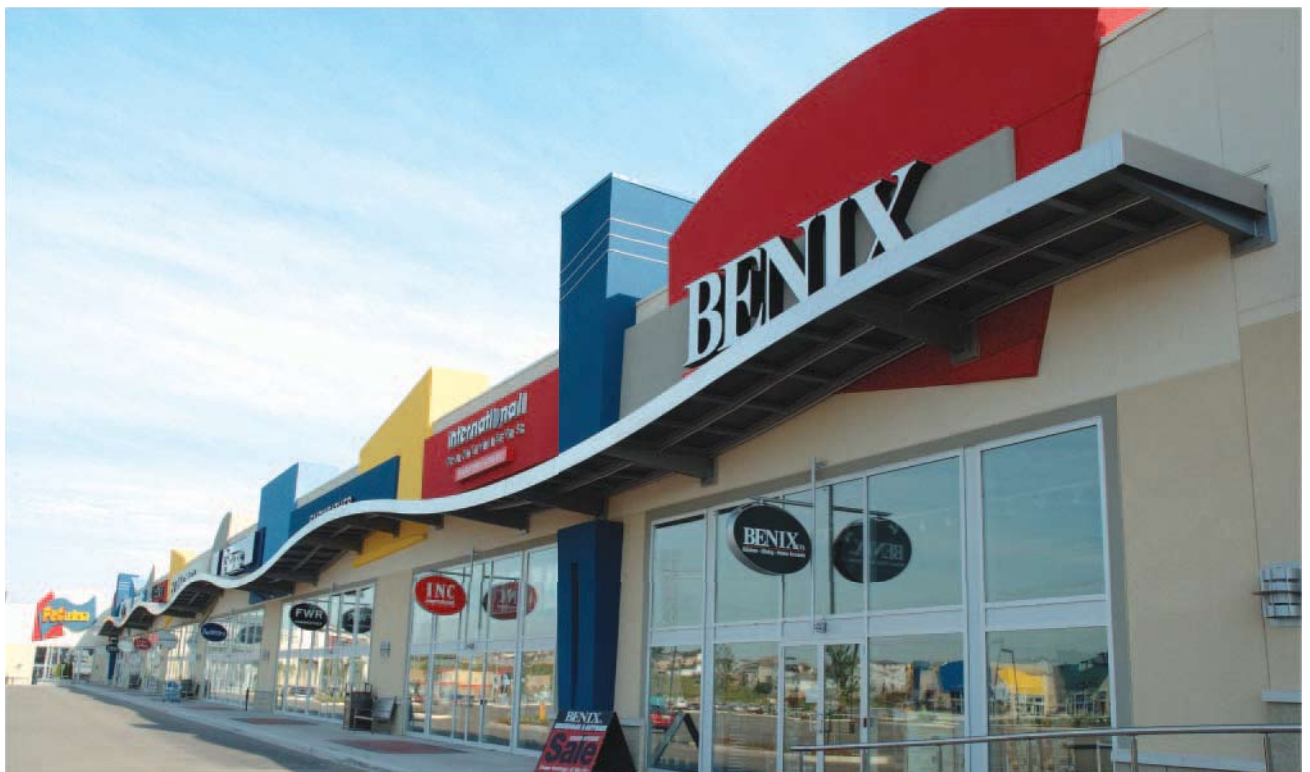
Seamless integration of canopy to multiple building surface planes
