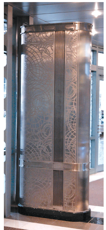
Custom stainless steel clad air supply tower
