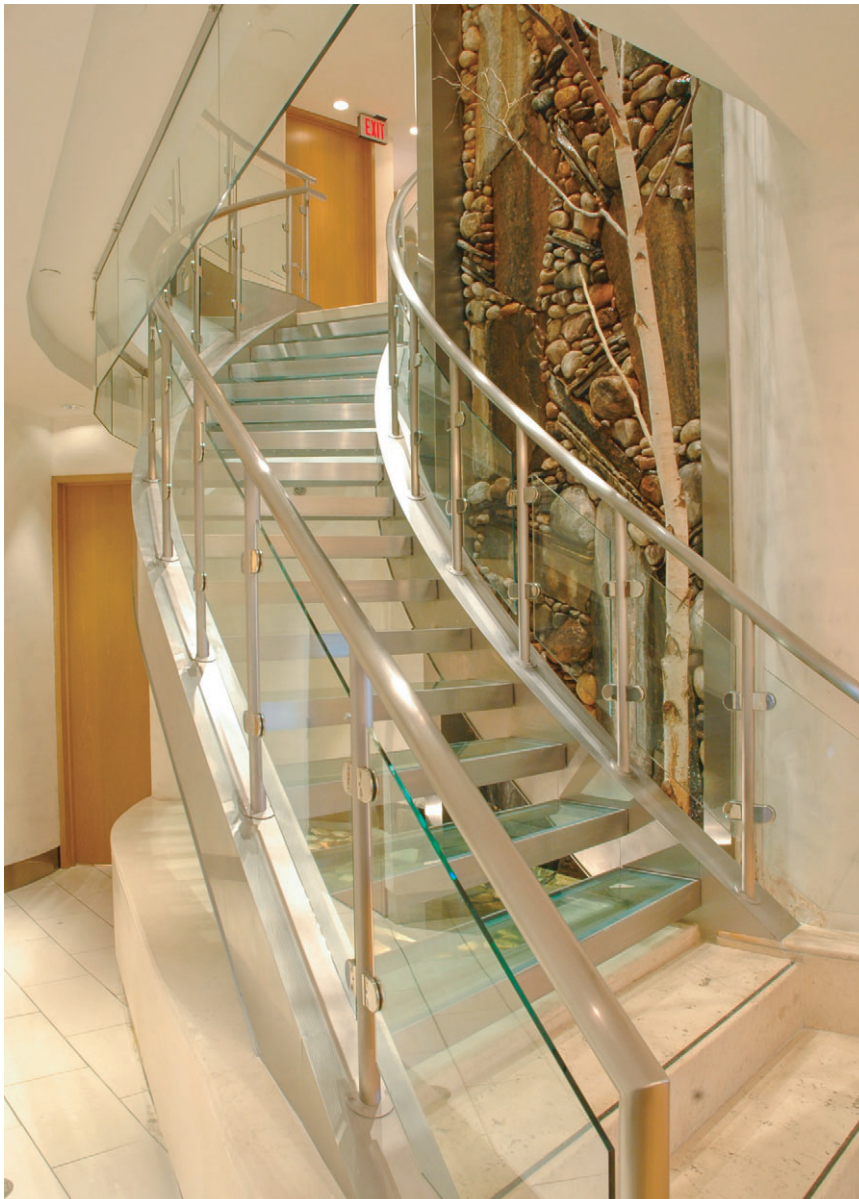
Monumental stainless steel staircase features five different curve radii, glass treads and glass panels
