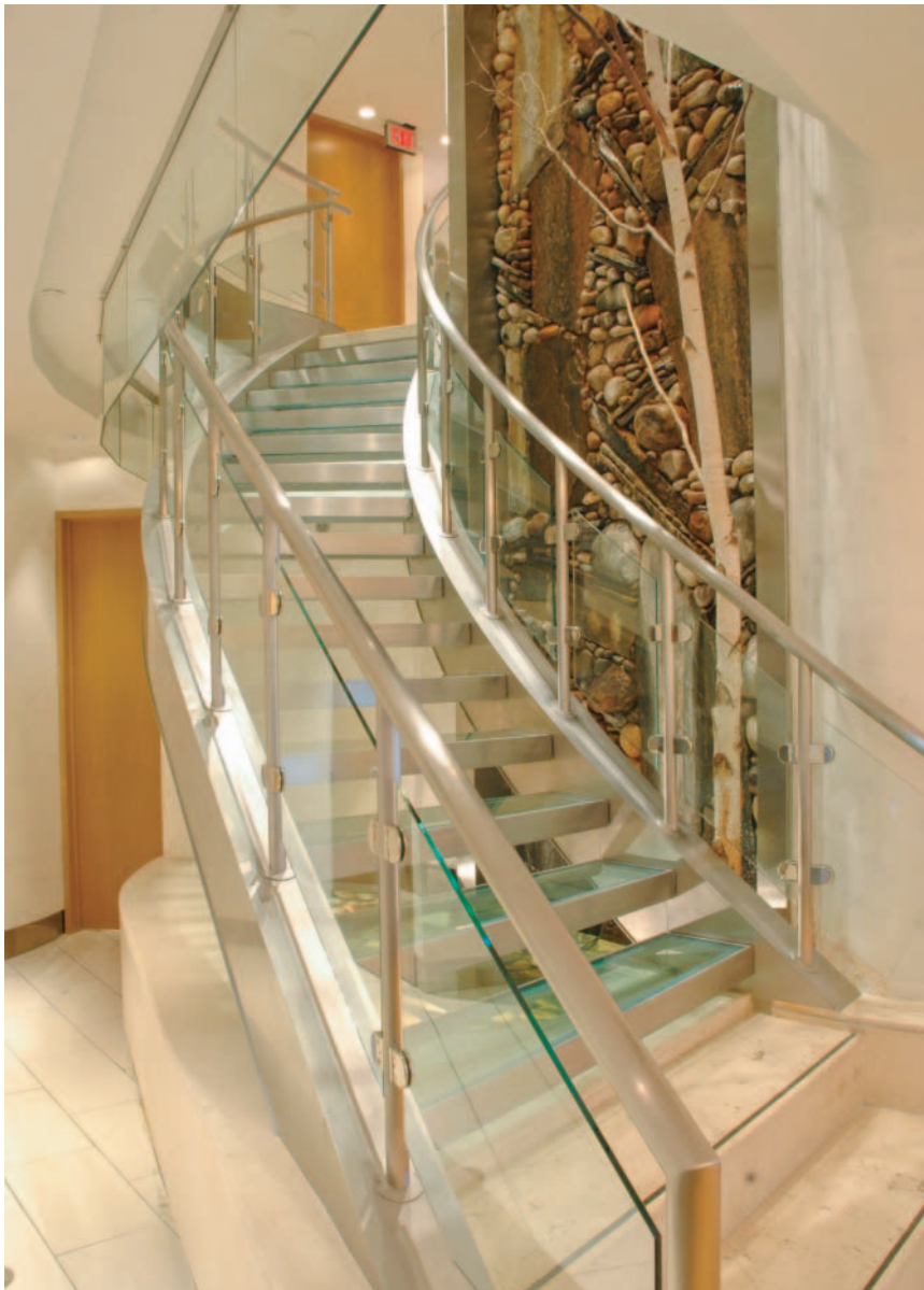
Monumental stainless steel staircase features five different curve radii, glass treads and glass panels
