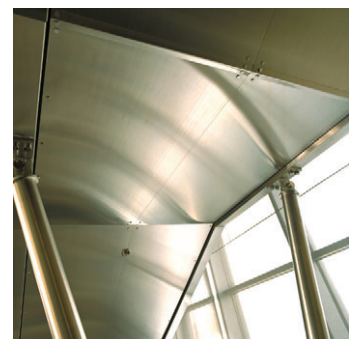
Cladded structural steel
