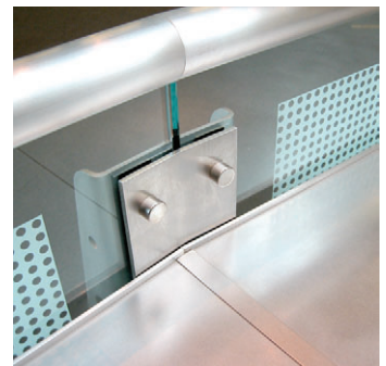
Modern fasteners and framing
