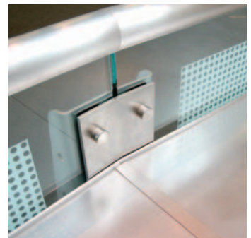
Modern fasteners and framing
