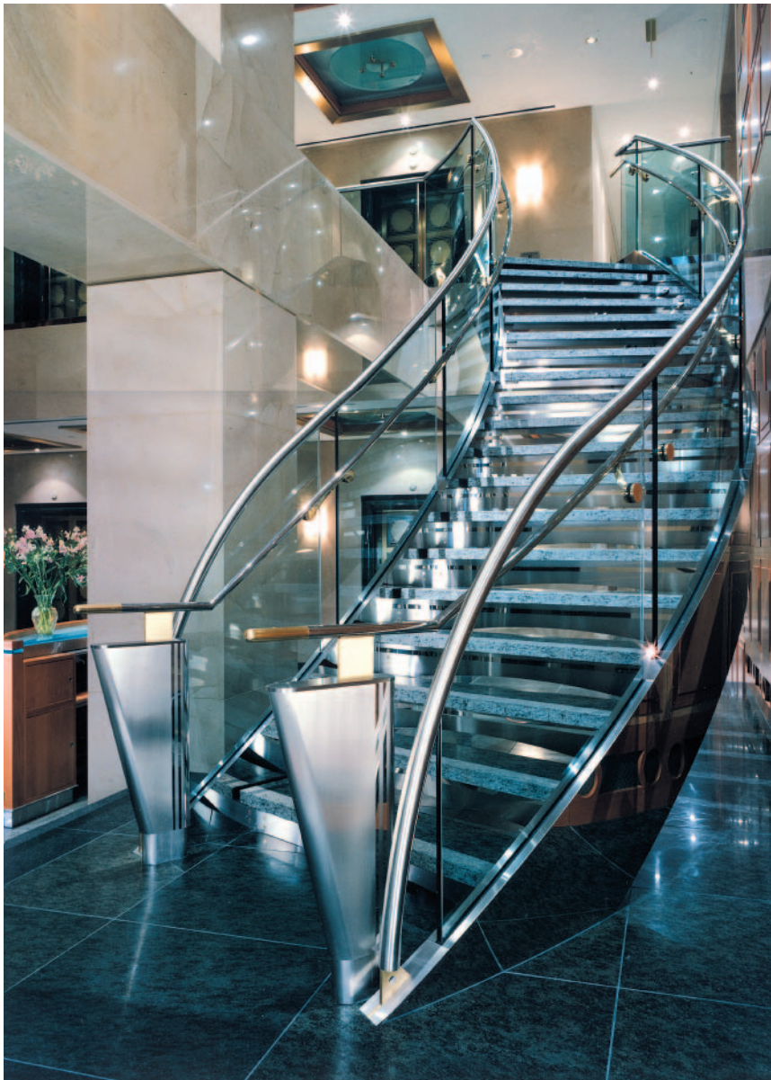
Monumental st. stl. staircase with mirror polished st. stl. stringers and guardrails and curved tempered glass
