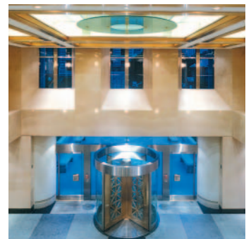
Brass framed ceiling lighting and st. stl. revolving glass doors
